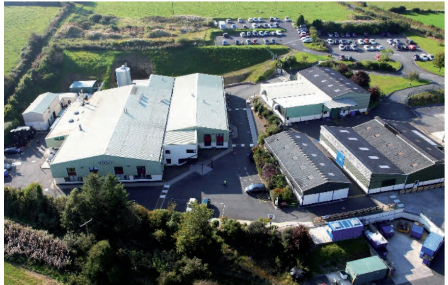
Aerial view of SERB's biologic manufacturing site in Wales. ©SERB
